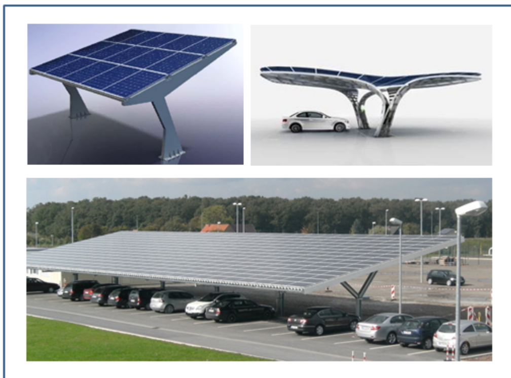
Figure 44: Different solar carport designs 62
