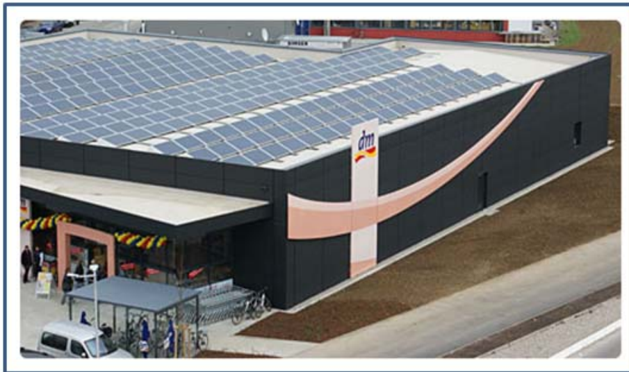
Figure 66: Roof-mounted solar PV at dm in Germany 85
