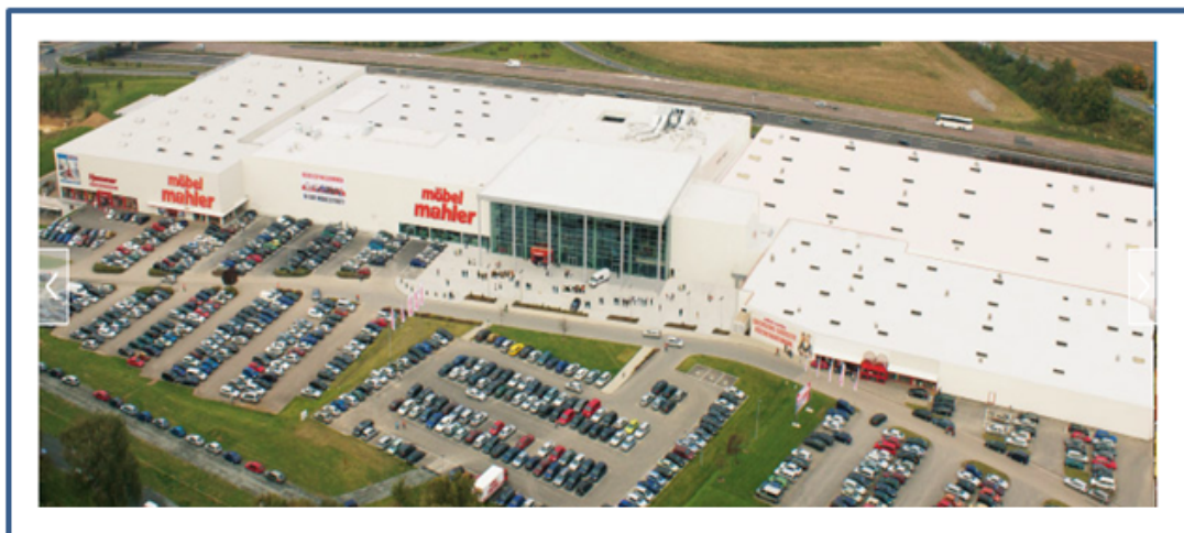
Figure 69: Typical opportunity for PV carport implementation 87
