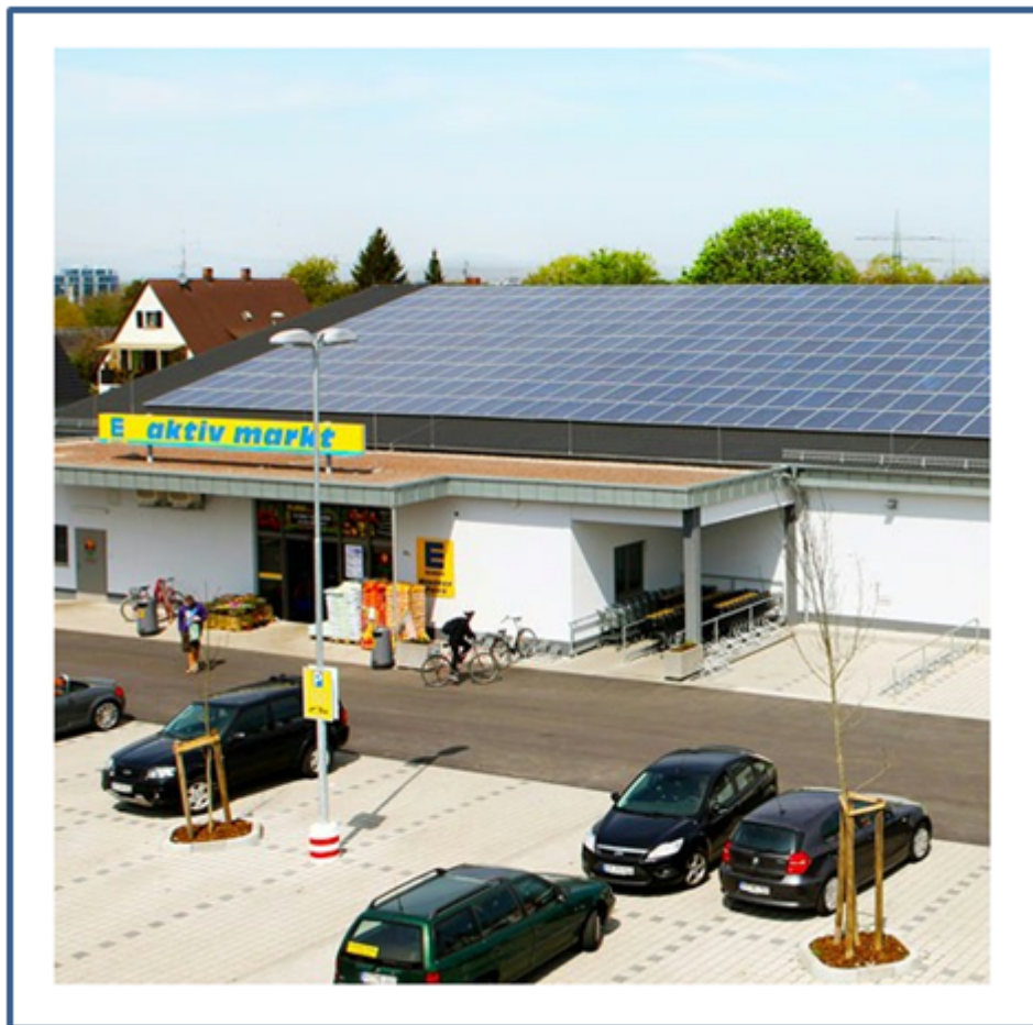
Figure 65: Roof-mounted solar PV on an EDEKA shop in Germany 84
