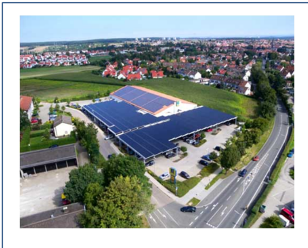
Figure 40: PV Carport at the EDEKA-Supermarket in Krawczyk 53
