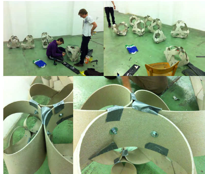
Fig. 3.75 First modules put together (top); tape was used to keep the components together until they were fixed with screws and washers (bottom).
