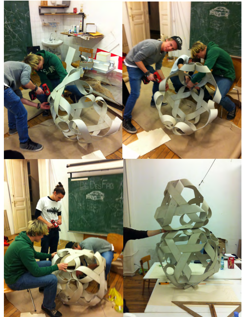
Fig. 3.56 Assembling one octahedron (top); the first two joined modules, one inscribed in a tetrahedron and the other one in an octahedron (bottom).
