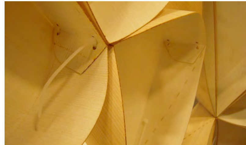
Fig. 2.13 Three cells joined with a zip tie.
