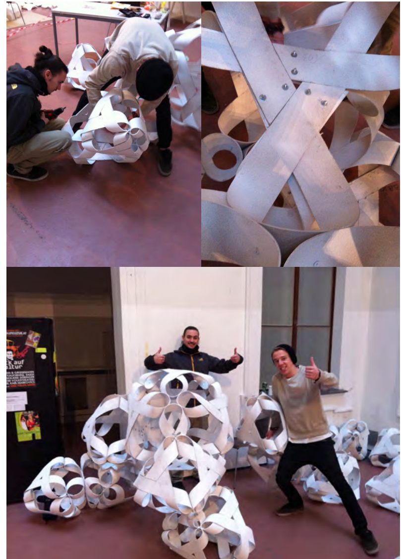
Fig. 3.79 Site assembly. Detail of two modules fixed with six screws (top right).
