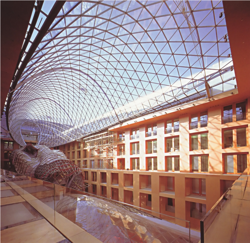
Figure 3.7 Triangulated glass roof in the DG Bank (2001) in Berlin, Germany, by Frank Gehry (Gehry, 2001, p. 219).
