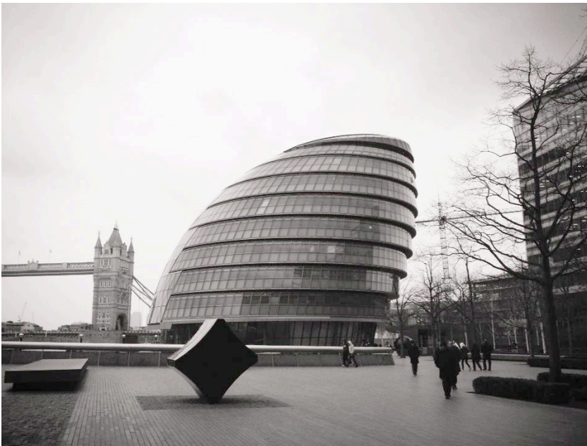
Figure 4.24 City Hall (2002) London, UK, architect Foster + Partners (© Reza B. Assasi 2013).
