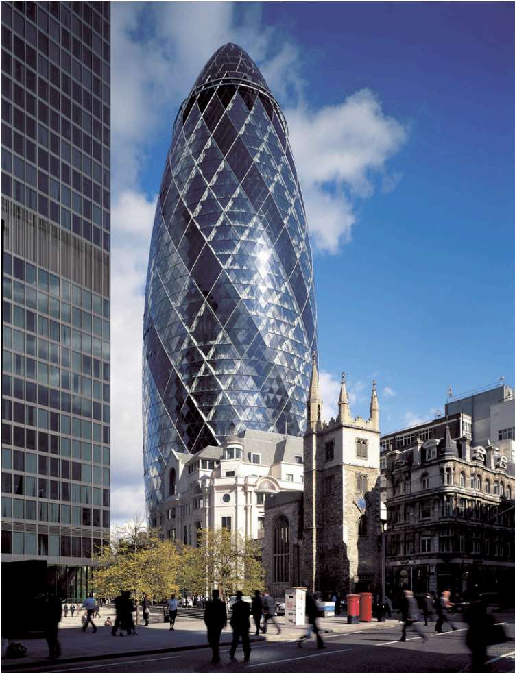
Figure 4.20 Swiss Re (1998), London, England, architect Foster + Partners (Young, 2004).
