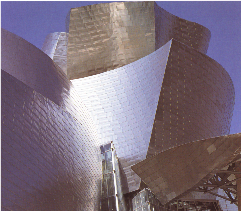
Figure 4.40 Implications of the geometric properties of developable surfaces on the aesthetics and construction of a design at the Guggenheim Museum (1997), Bilbao, Spain, architect Frank Gehry (Gehry, 2001, p. 170).
