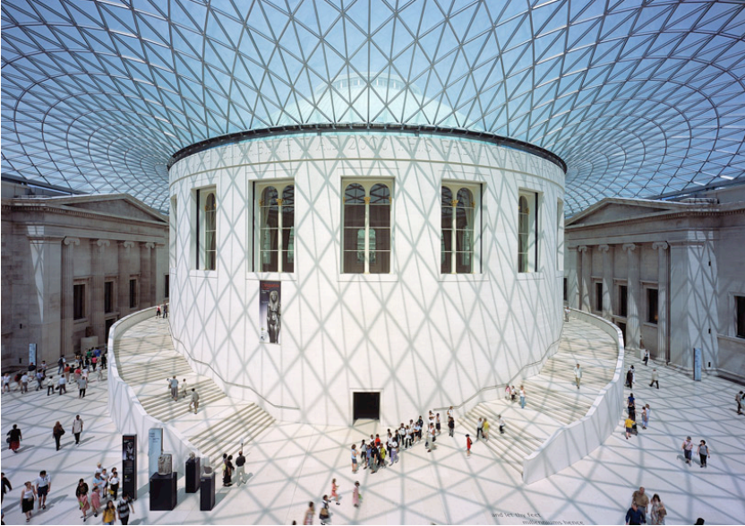
Figure 3.9 Triangulated glass roof structure in the Great Court in the British Museum (2000), London, UK, by Foster + Partners (Young, 2004).
