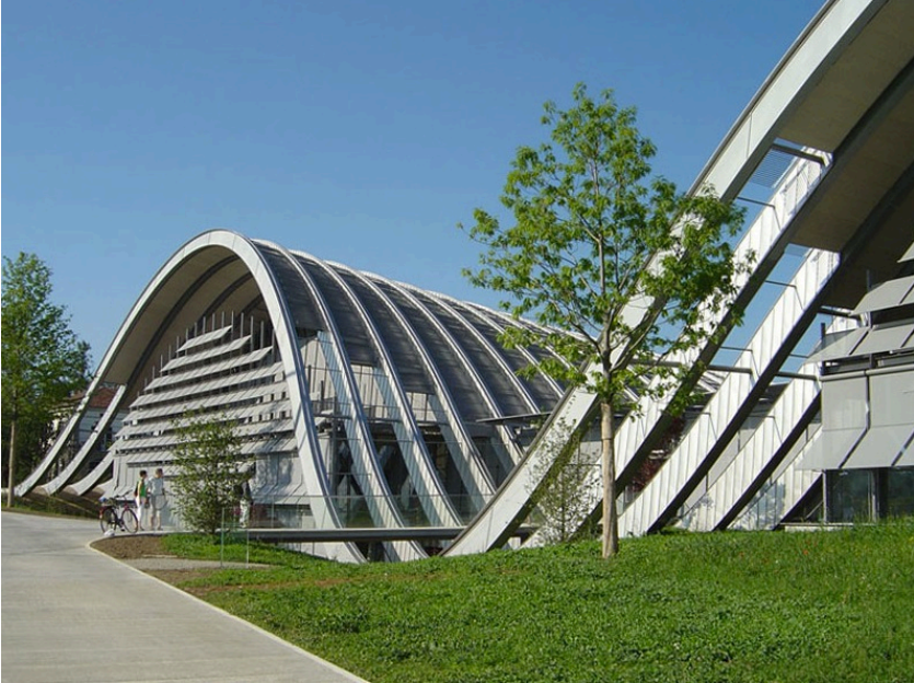
Figure 3.27 Zentrum Paul Klee (2004) in Bern, Switzerland, by Renzo Piano Building Workshop (Walz, 2012).
