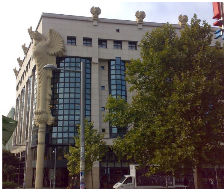
Figure 2. Vienna University of Technology Library, Resselgasse 4
