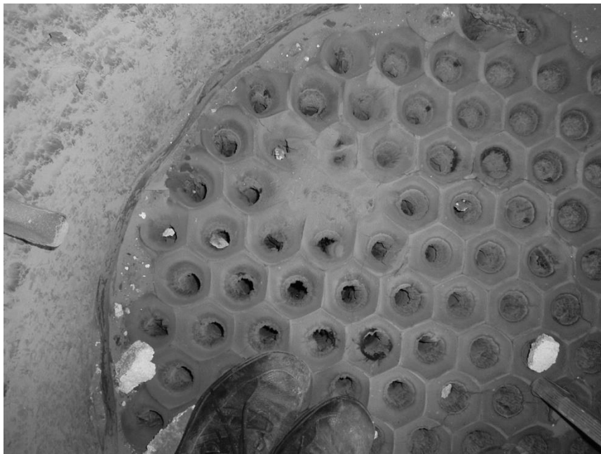
Figure 23: Fouling at the air preheater – view from the top at the tube sheet on the flue gas side
