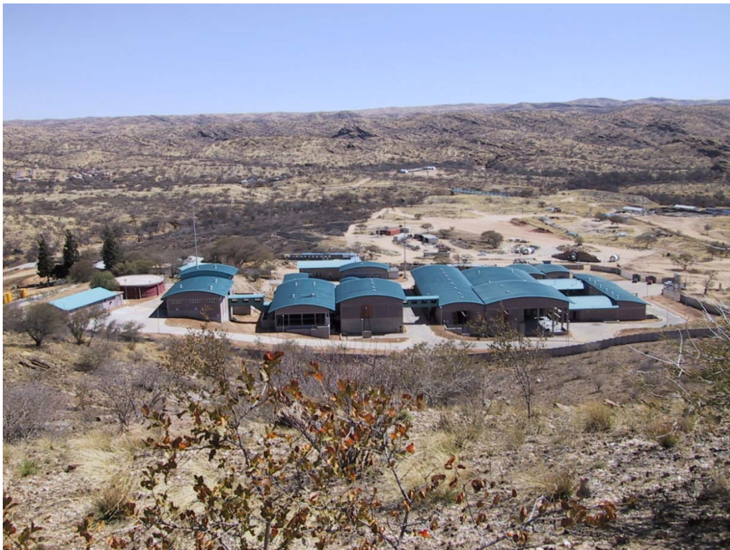
Abbildung 7: New Goreangab Water Reclamation Plant
