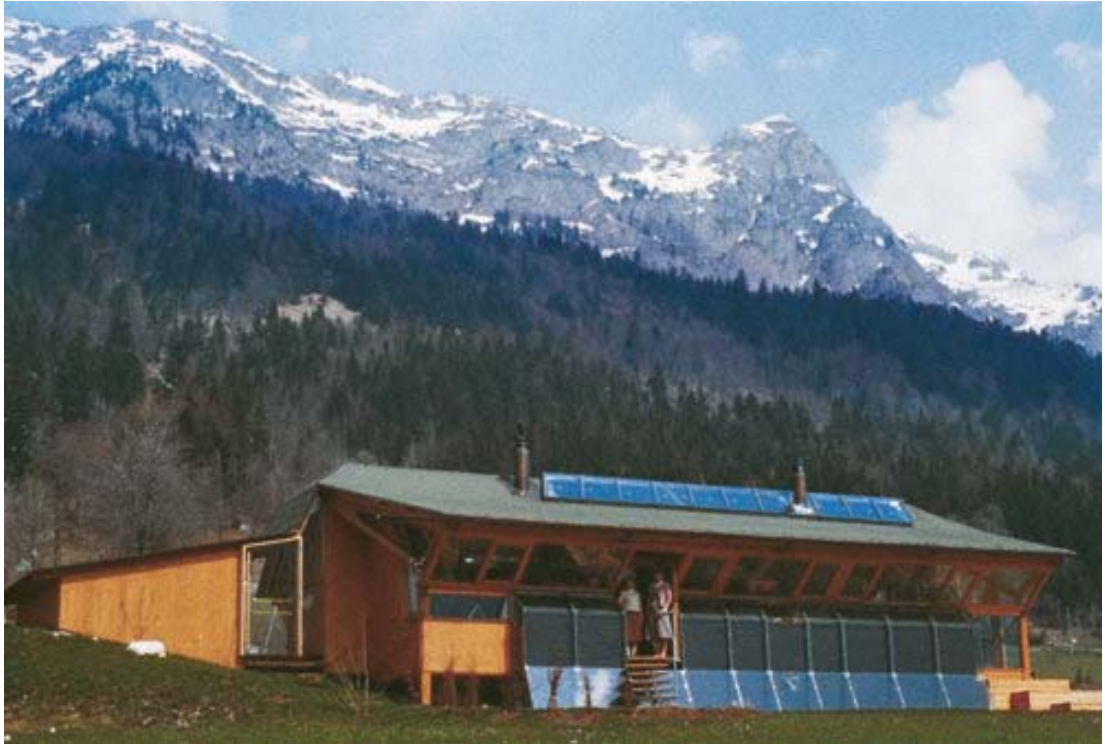
Figure 1-2 External view "Haus Fischer" Grundlsee, 1975-77 (source: Nextroom 2017)
