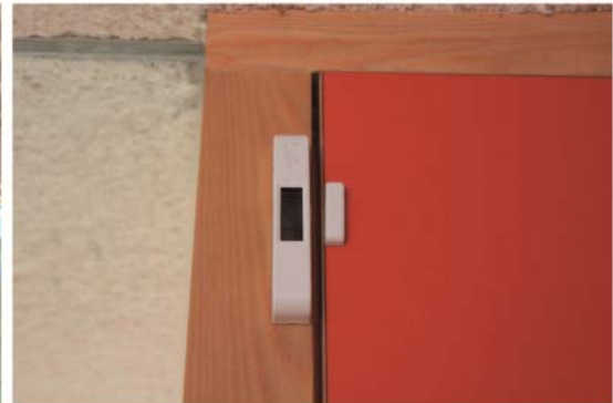
Contact sensor, door to corridor, Thermal Zone 6, #CA6
