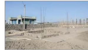
When I first arrived in Logia only the foundation of the hostel building existed. It was made of stones and concrete to achieve a better water protection of the earthen wall.
