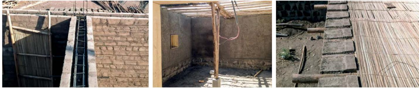
fig. 95: Ring beam with reinforcement before filled up with concrete
