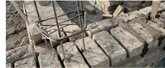
fig. 92: Hoops prepared for transverse reinforcement in every third row of bricks
