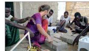
The system works like this: we always have three blocket, and in the middle we have one to maximum two centimetres hole here." It is important to always cover the joints with the next row of bricks.
