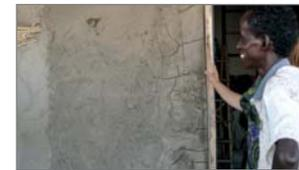
With three parts of sand and one part of soil there were still cracks. The best result we had was with a mixture of 4 parts sand and one part soil.
