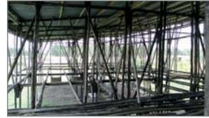
**Scene 39:** On the construction site of NESTown-project, it was easier to protect the bricks from rainfall, because the roof of the rainwater units had been constructed before the wall.
