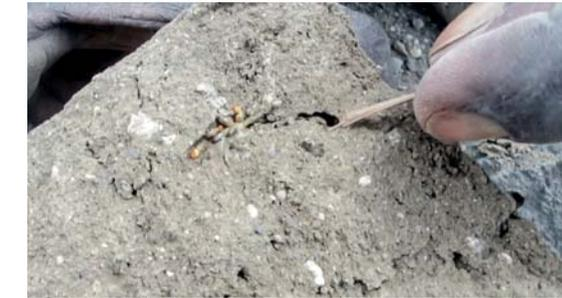
fig. 117: Breaking brick infested with termites
