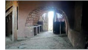
**Scene 43:** In SRDU-project, another construction for the ceiling was used; a vaulted ceiling, made of adobe bricks.
