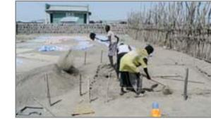
The soil comes directly from the building site. After removing the first five to ten centimetres of impure soil you can use the material underneath for brick production.
