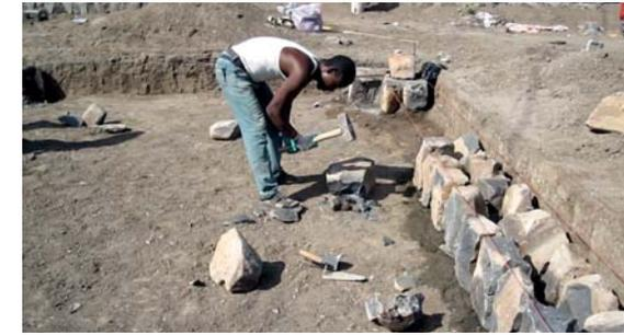
fig. 91: Mason hewing rocks for first section of foundation
