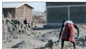
**Scene 28:** The reason for the shrinkage is the high amount of clay in the soil material. To reduce shrinkage and avoid cracks in adobe bricks we added sand as a stabilizer.
