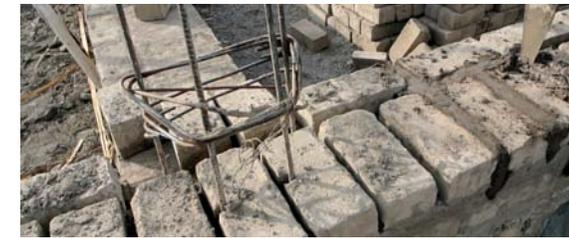
fig. 92: Hoops prepared for transverse reinforcement in every third row of bricks
