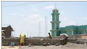
**Scene 6:** The finished air dried bricks were used to build up the wall. Adobe construction is a sustainable building technique that you can use in many regions of the country.
