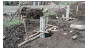
Because of the highly expansive black cotton soil, it is necessary to make a pile foundation. Then the wooden framework and the roof will be erected.
