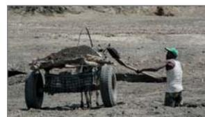
After the roof is finished the plaster will be prepared. It is made of soil coming from the riverbed. Straw is used as a stabilizer instead of sand. The mixture has to soak for about one week.
