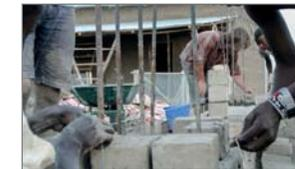
A tube filled with water is used to control if the corners are in the same height. Once two opposite corners are placed, a line will be fixed on them to enable straight masonry.
