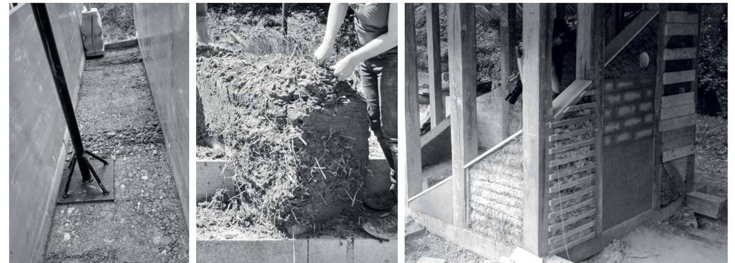
fig. 15: Rammed earth wall under construction
