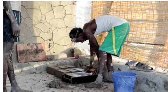
fig. 105: brick proction with a three-compartments mould
