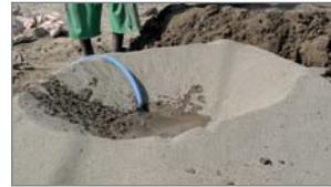
Sand and soil have to be mixed in dry conditions. Then a pile is formed with a hole in the middle that is filled with water. By shovelling the material into the middle, it gets mixed.
