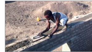
After 17 rows of bricks the ring-beam was constructed. Like the lintels, it was also made of reinforced concrete.
