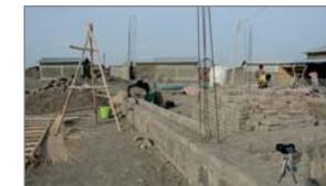
**Scene 36:** One row of bricks is composed of headers and stretchers. If the edge of the brick is visible on the surface of the wall it is called stretcher, if the end is visible header.
