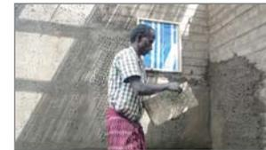
On the inside, the wall will be plastered with 2 layers. To enable a good adhesion for the second layer, we made notches into the moist plaster. On the outside walls there will be three layers of plaster.
