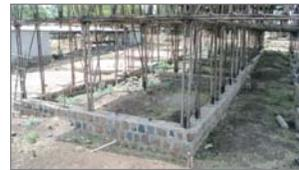
The adobe bricks will be placed between the studs, so they are only self-load bearing. Starting in the corners, one row of headers is followed by three rows of stretchers.
