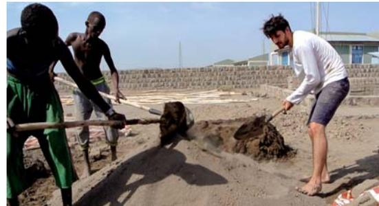
fig. 103: Mixing sand and soil in dry condition
