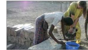
When the brick is in the right position, you have to push down strongly until a bit of the mortar comes out on the side. Katharina Schönher: "The pressure has to be to hold the brick and the mortar together, okay?"
