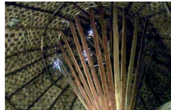
fig. 204: Holes in the bamboo roof of Adena SRDU
