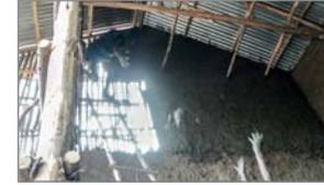
The inside of the house will be plastered first. The outer protection can be either made of mud or cement plaster.
