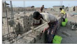
The joints need to be filled from above with mortar. Every third row a transverse reinforcement was installed additionally. The hoops were bent by hand.
