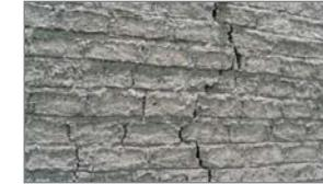
In particular, the relationship of mud bricks to water needs to be clarified. Walls got damaged because they were not protected with plaster and bricks were left outside without covering them appropriately.
