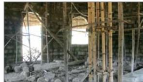
As this dwelling unit has not actually been finished, you can see the brickwork very well. Like in NESTown, a wooden framework and the roof have been constructed before the brick wall was erected.
