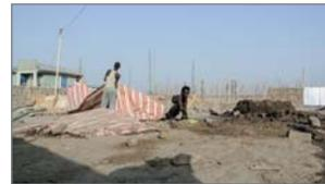
When the mixing is finished the mound needs to be covered with plastic and soaked for two to four days.
