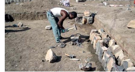
fig. 91: Mason hewing rocks for first section of foundation
