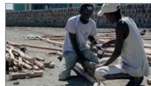
**Scene 47:** Finally it was time for the construction of the second floor and the roof. A part of the wooden framework had been pre-constructed on the ground.
