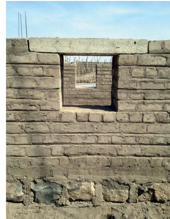
fig. 93: construction of a lintel
