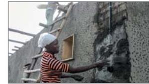
**Scene 42:** After the ring beam was finished it was important to plaster the wall, so it was protected from rain. We did some experiments to find the right mixture for the available materials.
