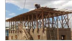
The roof was covered with corrugated iron sheets. A large roof overhang is good to protect the adobe wall from rainfall. The mud floor and the plaster were also completed.
