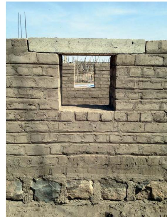
fig. 93: construction of a lintel
