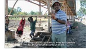
...with the format of 13 to 13 to 28 centimetres. With the single mould, you would need four people for the production of four bricks. But with the new mould, you only need two people to produce four bricks."
