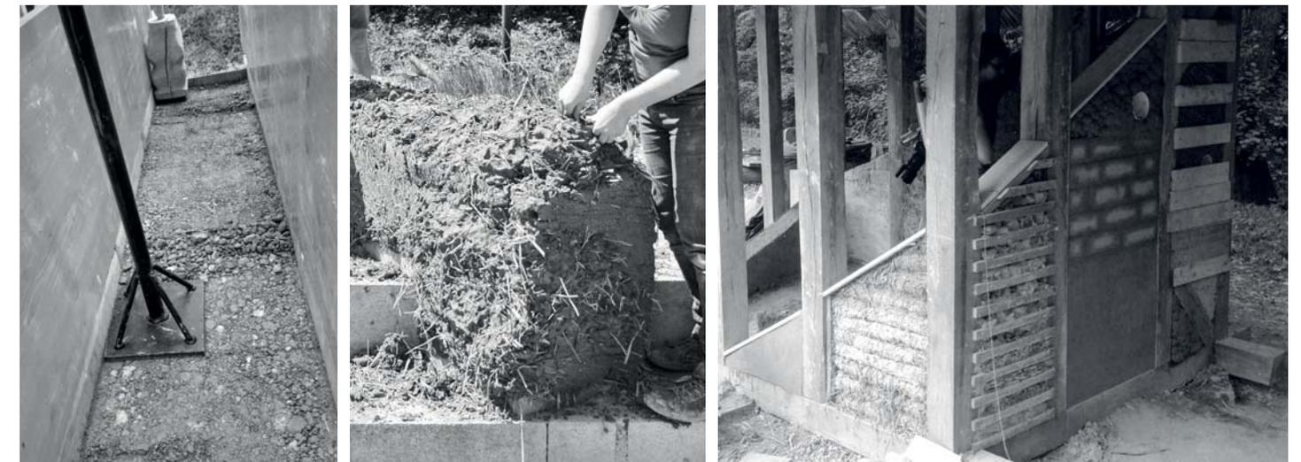
fig. 15: Rammed earth wall under construction
