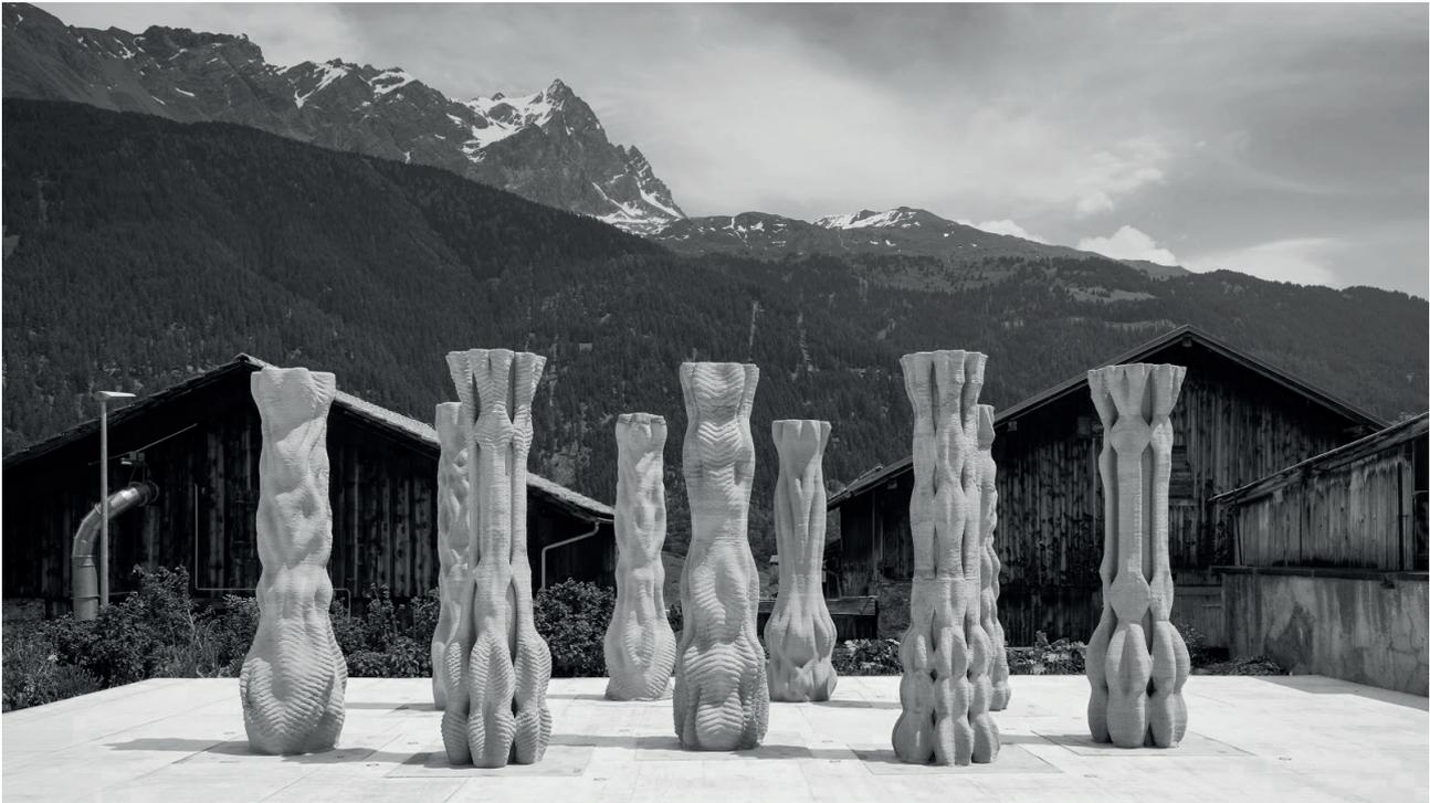
Fig. 1: Concrete Choreography: Nine concrete 3D-printed columns. Photo: Benjamin Hofer
