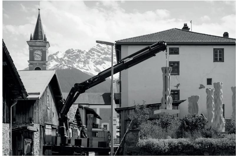
Fig. 5: Columns transported and lifted on-site in Riom, Switzerland. Photo: Benjamin Hofer
