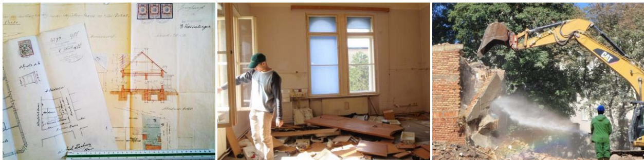
Figure 6 Analysis of plan documents, on-site investigation, and analysis during the demolition.
